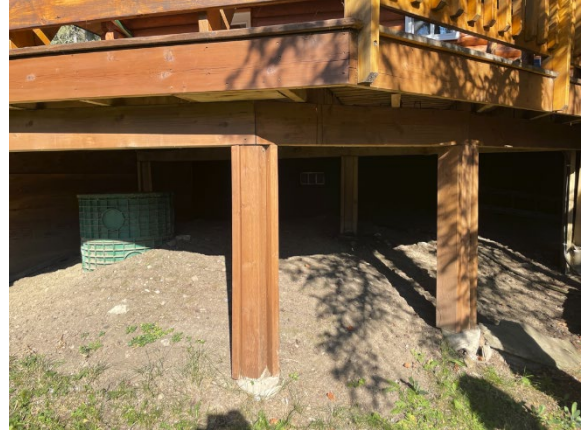
Removal of combustible debris and vegetation under decks
