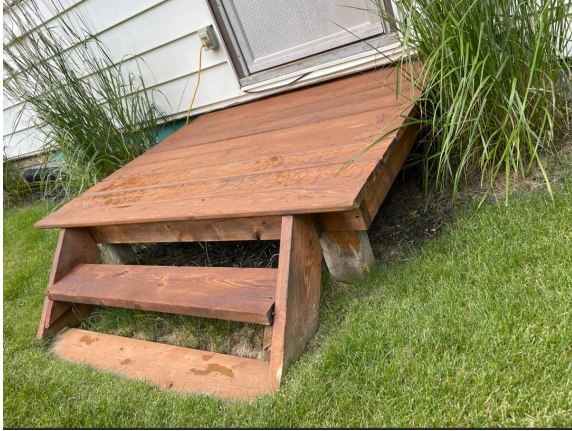
Replacement deck boards that were rotten or contained large cracks
