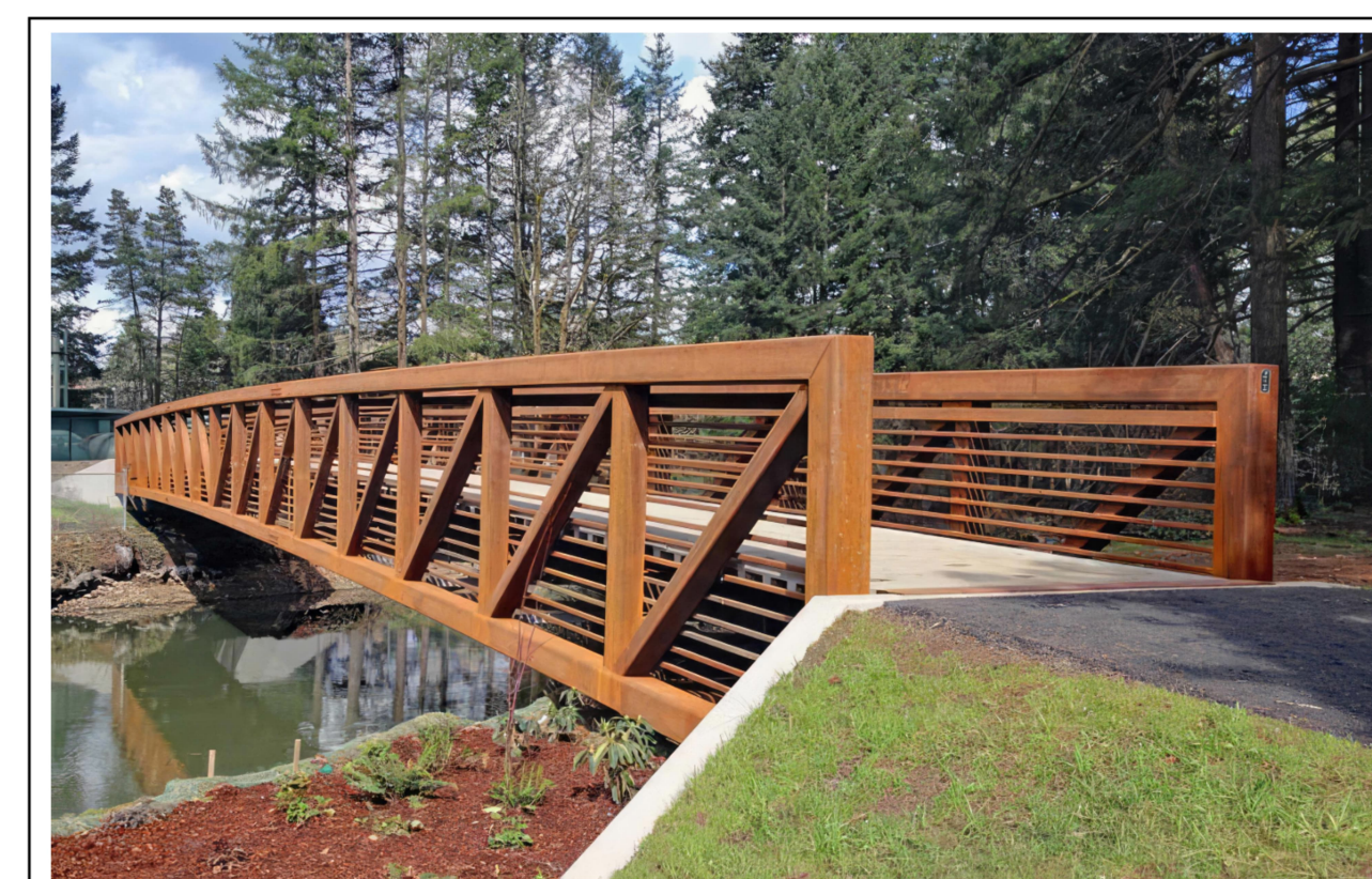
Pedestrian Bridge, Example 2
