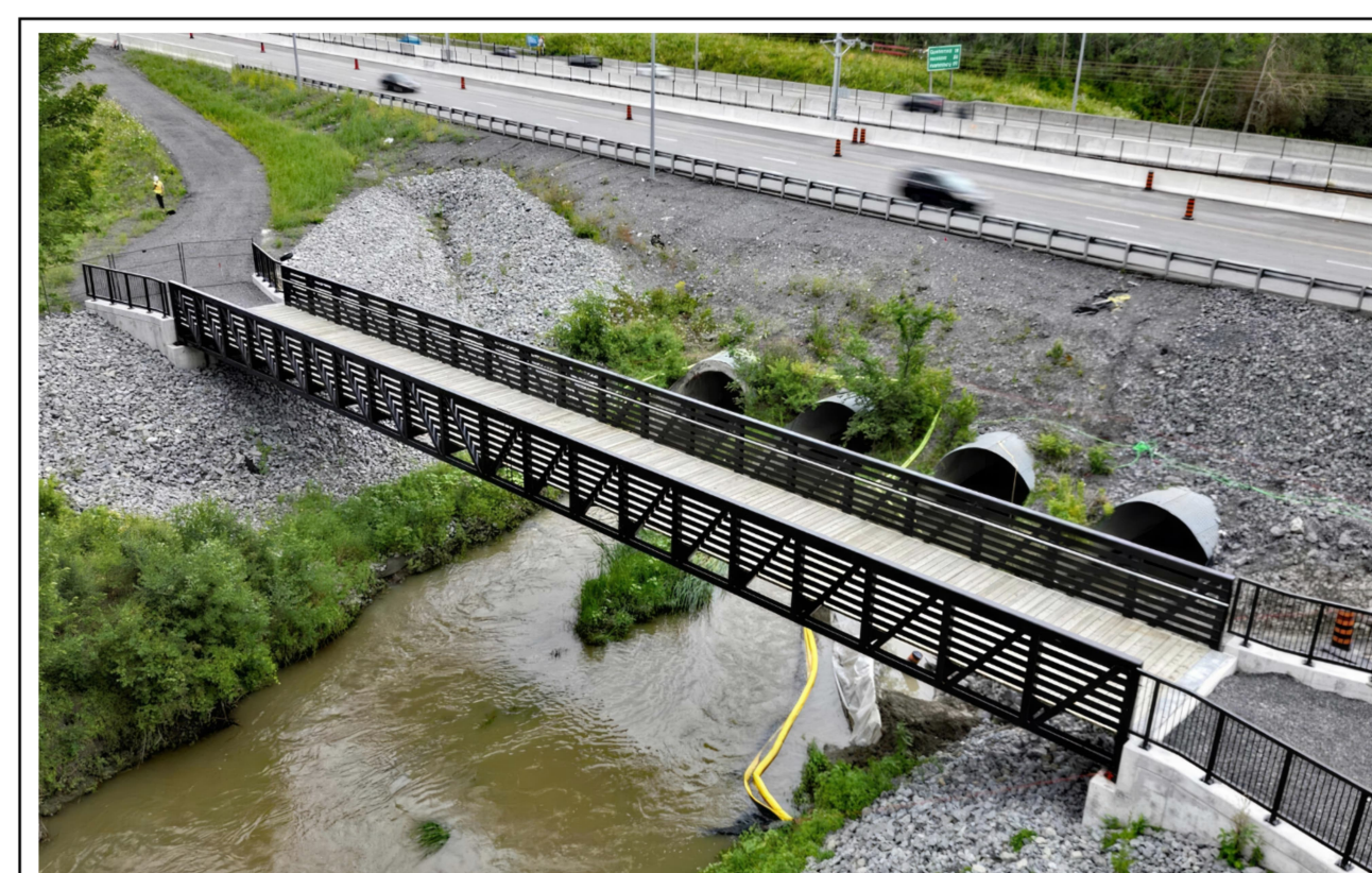
Pedestrian Bridge, Example 1
