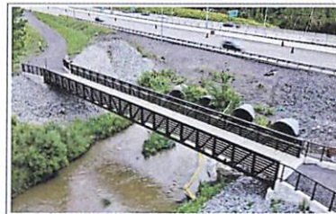
Pedestrian Bridge, Example 1
