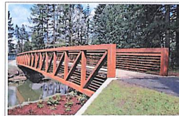
Pedestrian Bridge, Example 2
